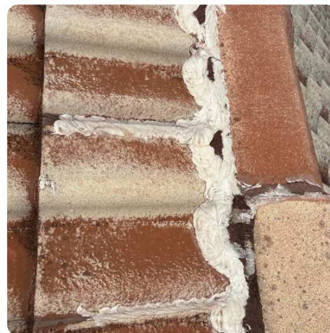
Sealant applied to hip capping bedding and tile laps adjacent to the party wall
