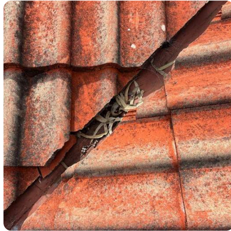
Organic matter trapped in valley beneath tile edges
