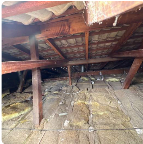
Roof space showing under purlin, struts and flue penetration, tiles unsarked
