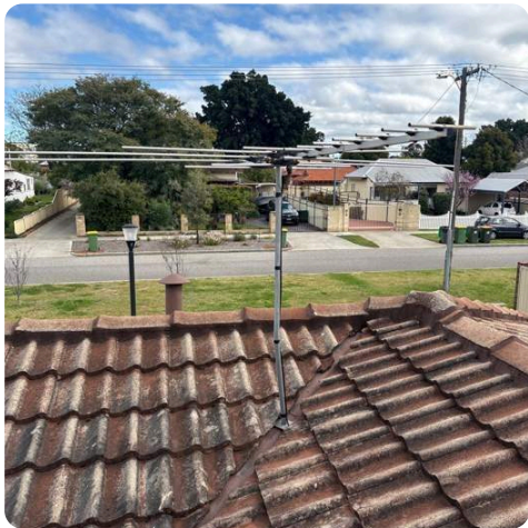
TV antenna mast mounted in the valley flashing
