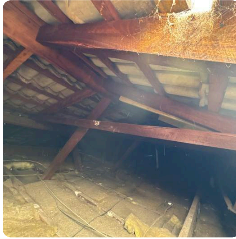
Under purlin and strut with a pine packer fitted between purlin and rafter
