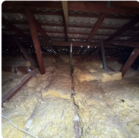
Roof space, timber framing and insulation, daylight visible through tile laps
