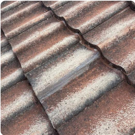
Second silicone sealed tile above the other living area ingress zone
